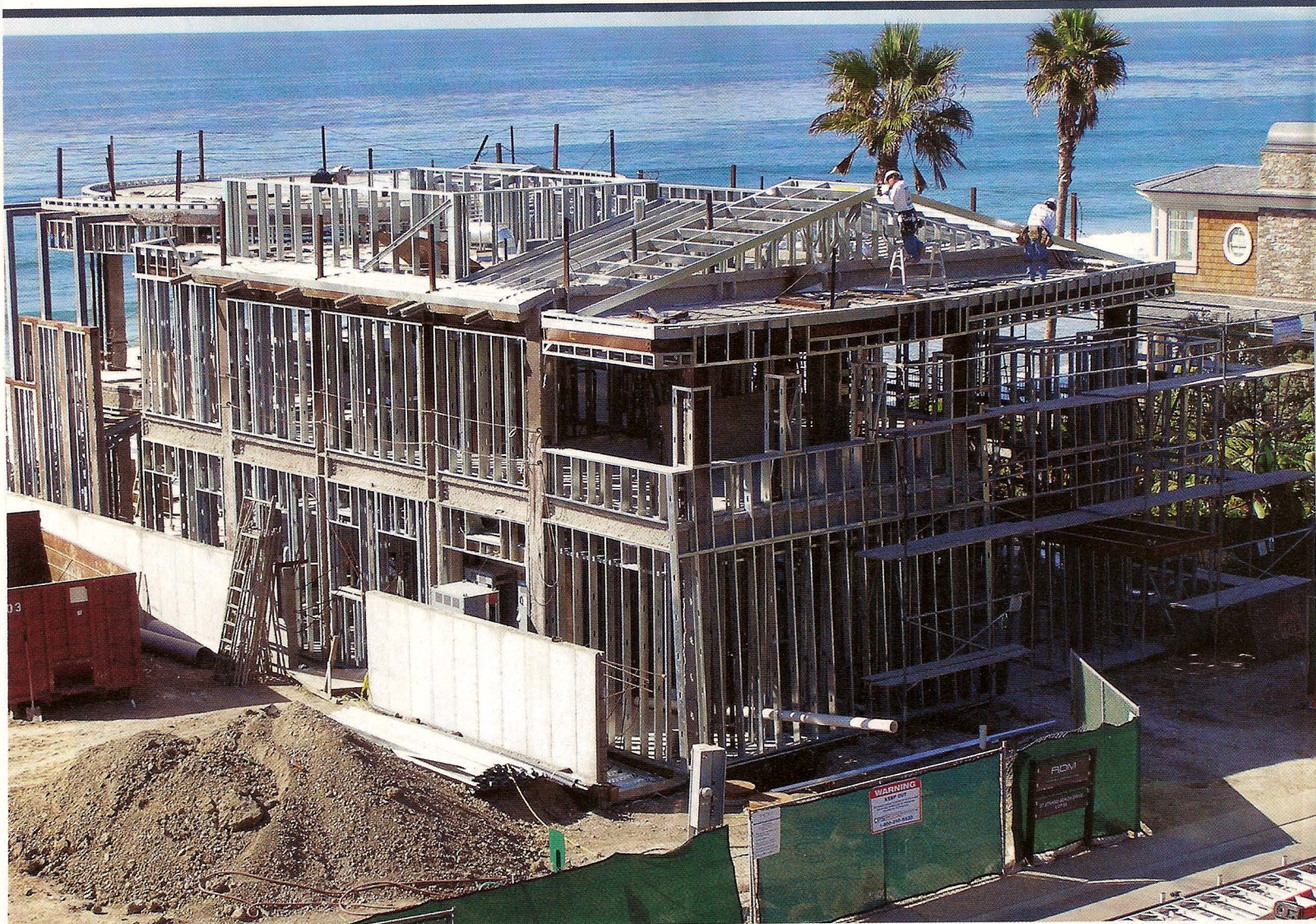
Steel framing on residential construction has gained greater acceptance in the custom home building market than with production builders, providing greater design flexibility and improved performance over wood.
